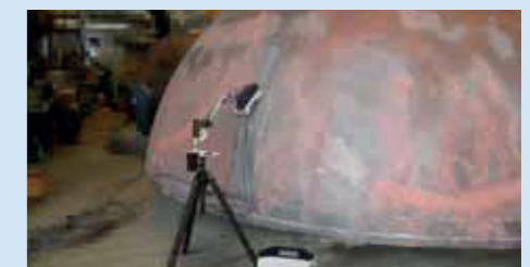
Storage tanks : Weld and annealing effects
